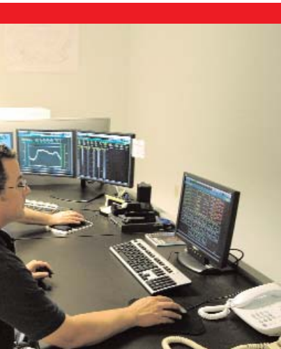
Allegheny Electric Coordinated Load Management System technicians Jim Line, Mark Bublinec, and Matt Shaud, left to right, monitor electricity demand and weather conditions 24 hours a day from a master center located at the G&T’s headquarters facility in Pennsylvania.
